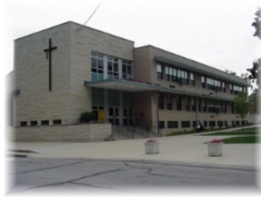
Jr. High Building
